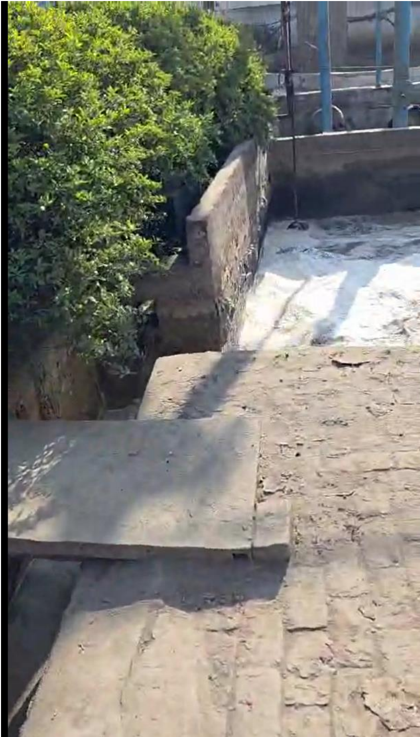
After Hill Screen effluent reaches Equalisation Tank
