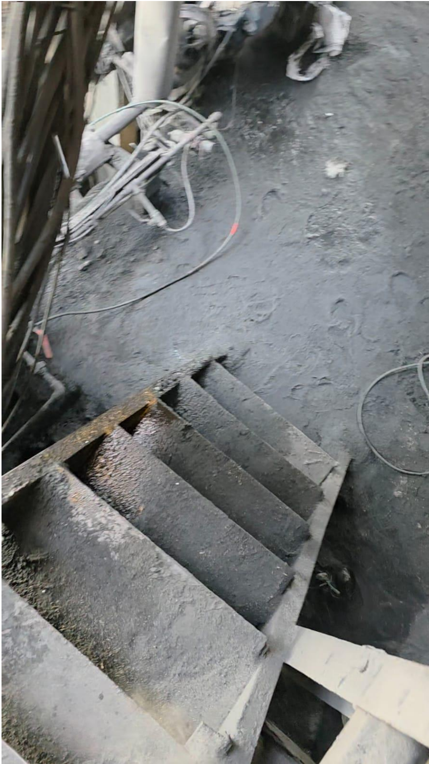
Stairs down the boiler
