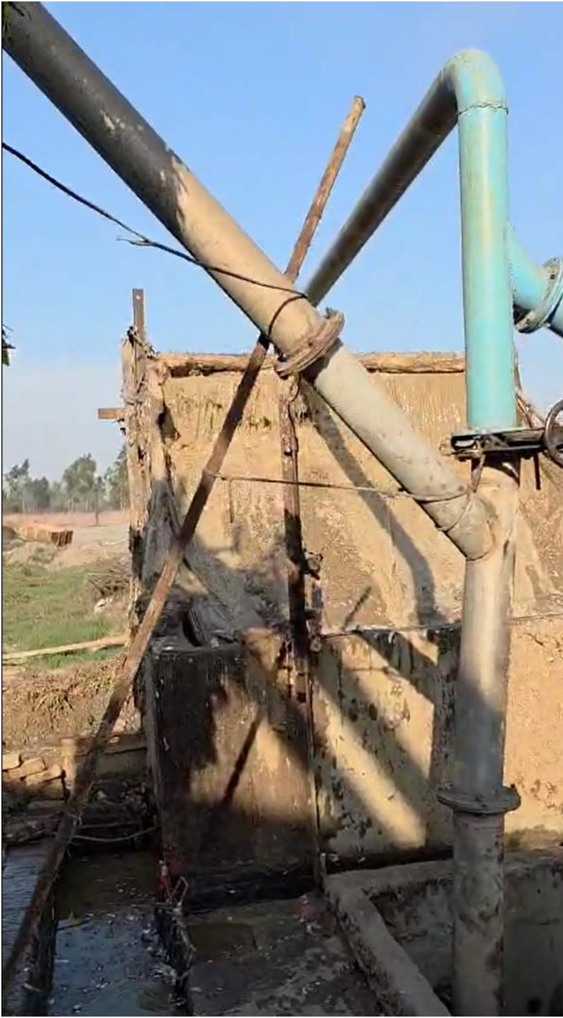
Hill Screen for recovery of materials for reuse.
